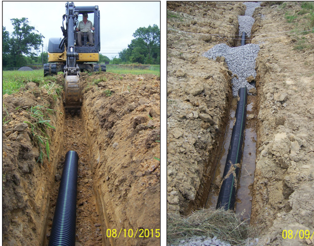
Trenching and backfilling an underdrain
