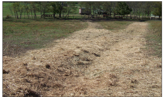
Seeding and mulching a swale
